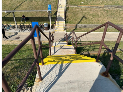
Stairs North Side
