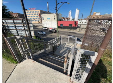
Ashland Stair Access
