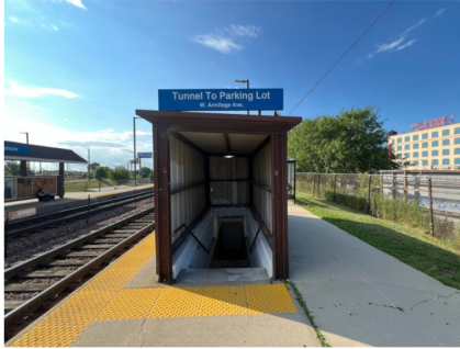
Station Platform Tunnel
