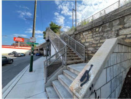
Ashland Stair Access
